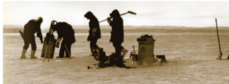
Radioactive debris being prepared for removal. In general, the materials were wrapped in plastic film to prevent dust or any other air-borne particles. The more radioactive elements were then manipulated into special shielded crates for safe transport.
