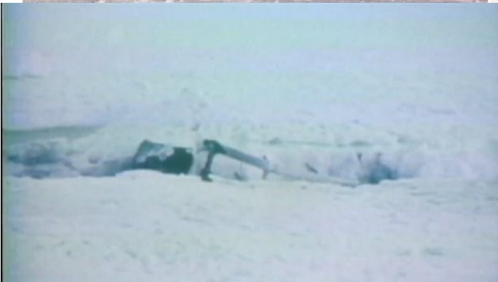
Radioactive debris being prepared for removal. In general, the materials were wrapped in plastic film to prevent dust or any dust or fine particles. The more radioactive elements were then manipulated into special shielded crates for safe transport.
